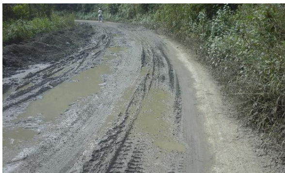
Figure 20:PAVEMENT CONDITION OF THE PROJECT ROAD
