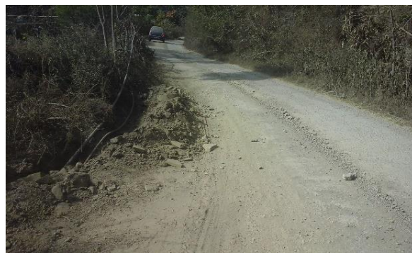
Figure 20:PAVEMENT CONDITION OF THE PROJECT ROAD
